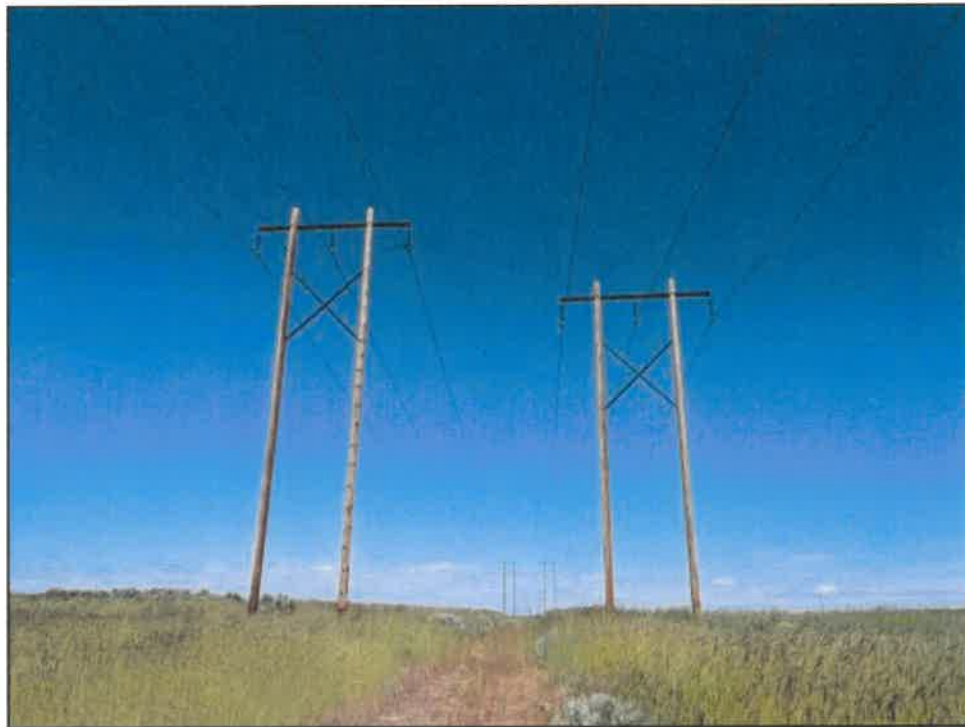
Figure 22. Representative image of conditions along the B-F transmission line corridor, showing B-F No. 1 H-frame tower #16-6 (right) and B-F No. 2 H-frame tower #16-6 (left) divided by a tow-track.
